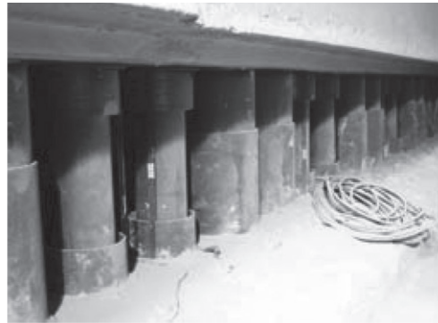
(b) Metallic slots in a test section of Lilla tunnel (Lower Ebro Basin)
